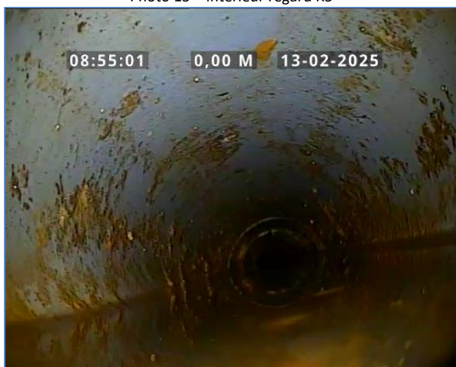
Photo 17 – Segment R1-R4 > pente insuffisante
